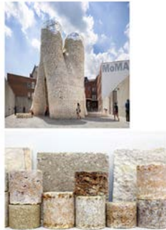
A 70 foot tower constructed with a selection of various shaped mycelium bricks
